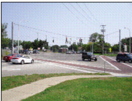
Street Level View of Intersection That Was Reconstructed With Precast Panels
