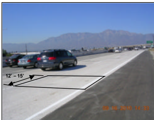
Non-Planar Panels Installed on An Apparently Planar Alignment
