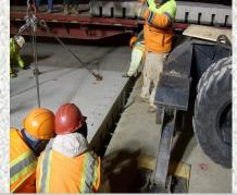
The project included repair of both two and three lanes of approach slabs for four bridges. Normal weight concrete slabs were 11-1/2" thick and 9-1/2" thick, separated by an asphalt pressure relief joint. Slabs were of variable length on horizontal and vertical curvature.
