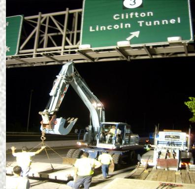
The project included restoration of 5.5 miles of this 6-lane state highway. Normal weight precast concrete Super-Slab® panels were used for full-depth replacement on the roadway. Work zone closures were generally limited to eight night-time hours during which two of three lanes could be closed for work.
