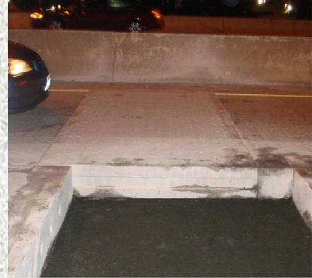
This first precast concrete paving project in Pennsylvania was installed in 8-hour night closure work windows in very restricted work areas in a depressed roadway section through the heart of downtown Philadelphia.
