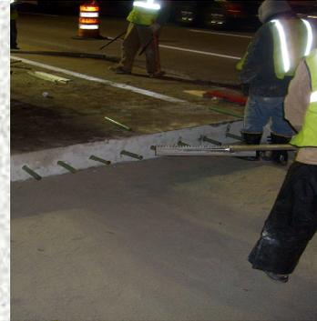
The project consisted of emergency pavement repairs to a gore area (between two travelled lanes) that had broken up and had become a danger to the travelling public. Slabs were installed in extreme cold weather and required special ground-thawing equipment for heating the slabs to cure the dowel grout and bedding grout.
