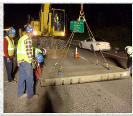
The project included restoration of 8 miles of this 6-lane Interstate highway. Normal weight precast concrete Super -Slab® panels were used for full-depth replacement on the roadway. Work zone closures were generally limited to eight night-time hours during which two of three lanes could be closed for work.
